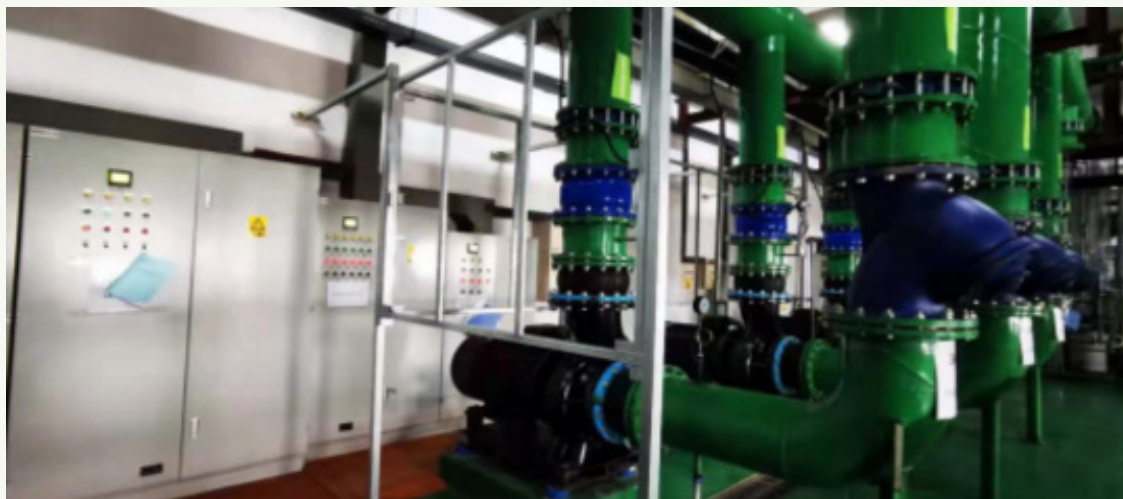
Frequency Conversion System of Air Conditioning Water Pump
